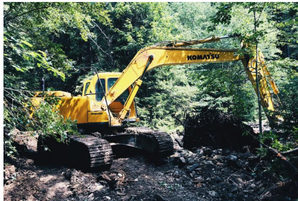
Big yellow digger clearing forest by a river © unsplash
