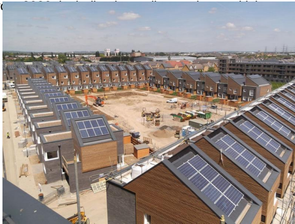
View of new housing development with solar panels © Ashden
