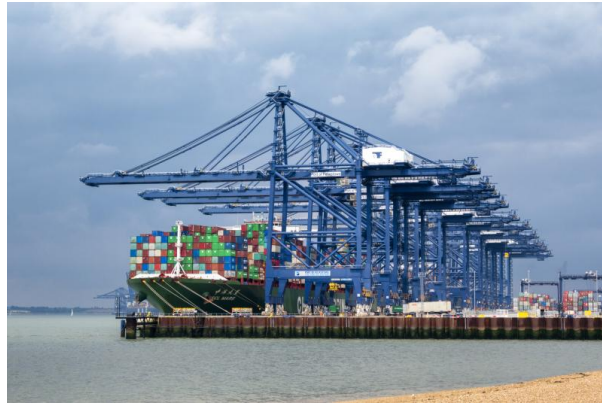
Container ship being unloaded at Felixstowe by giant cranes © iStock
