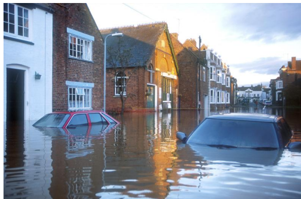
Submerged cars in flooded street in Bewdley, Bridgnorth © FOE EWNI/Paul Glendell
