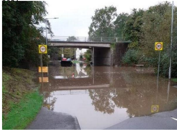
Flooded road, Heol Las in Swansea, October 2021 © Swansea Council
