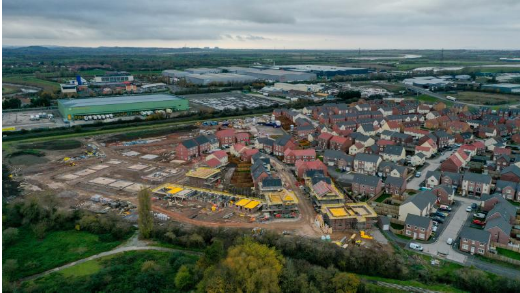
Aerial view of housing estate under construction, Bridgwater Somerset iStock
