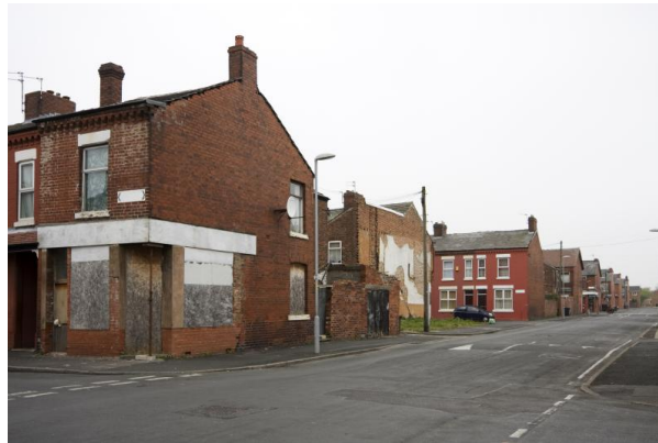
Houses in disrepair in Moss Side, Manchester © Getty Images
