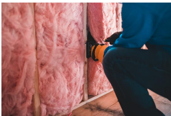
Man installing home insulation © Unsplash
