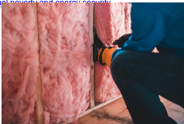
Man installing home insulation © Unsplash
