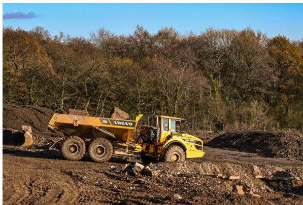
Dumper truck moving a load of soil on the site of a new housing development. © iStock
