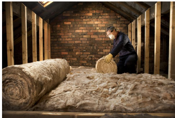
Installing loft insulation © Credit: sturti via Getty Images
