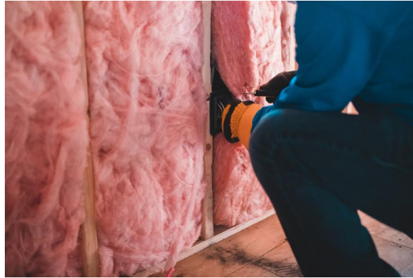
Man installing home insulation © Unsplash
