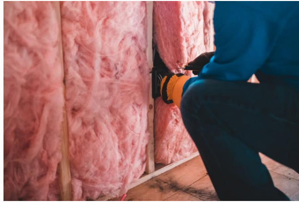
Man installing home insulation © Unsplash
